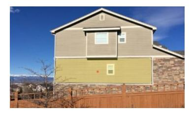
The edge lines of the siding and the frame can be used as guides for creating an alignment rectangle. Using these lines, create a large rectangle. It is better to have a larger rectangle than smaller, and also ensure that the rectangle encompasses the Spike laser (red dot).
